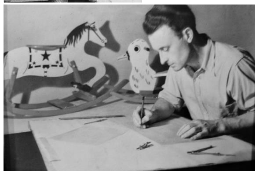
Leslie at his drafting table for the Delphos Bending Company courtesy of the Delphos Canal Museum
