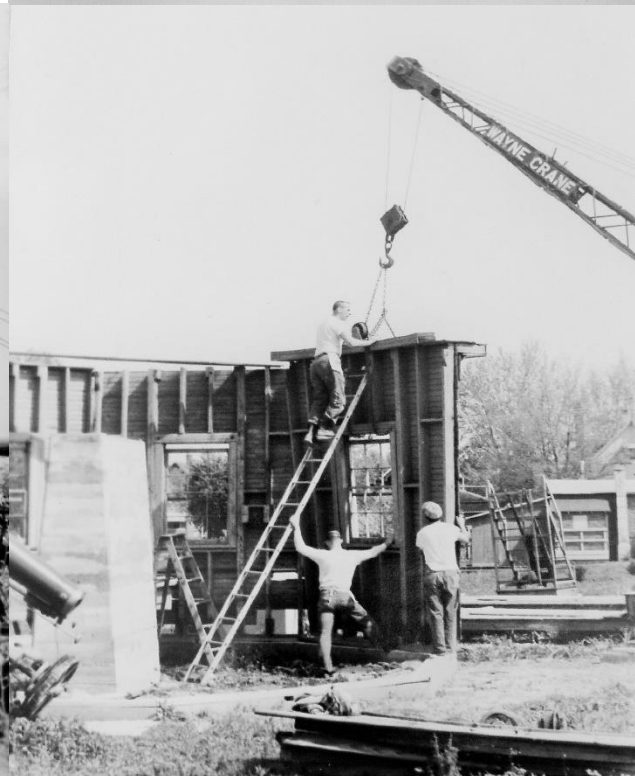
The telescope pier was placed in the meridian by aligning the concrete forms, at night, with two plumb lines set in line with the true north position in the sky.
