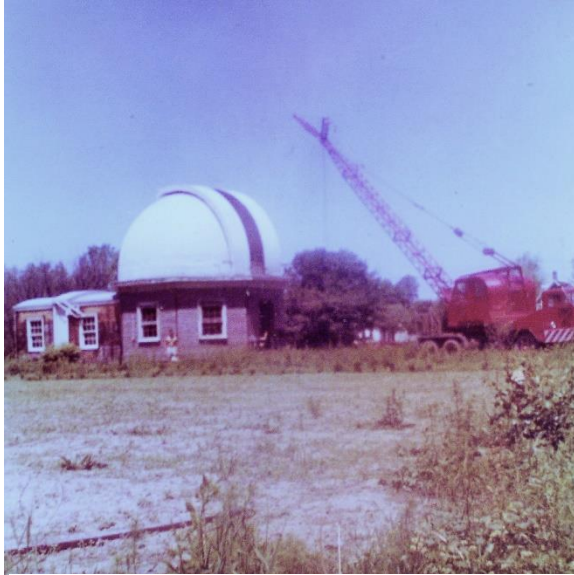
After the crane finished mounting the 22-foot dome
