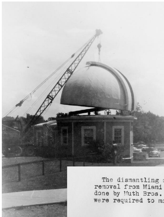
To transport the 22 foot dome it was necessary to saw it in half and then nest the two canvas and wood framed halves together to fit it onto the trailer.
